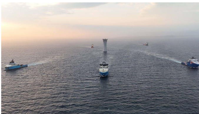
The Cenovus 210,000-tonne concrete gravity structure (CGS) on its way to the White Rose field area
