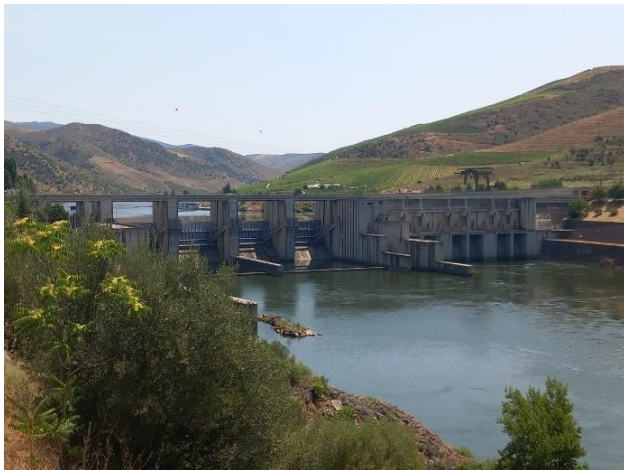
Pocinho Barrage and Lock on the Douro
