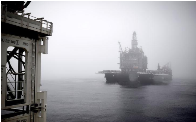
West White Rose - finally installed together, the Topside was mated to its CGS, and of course, it wouldn't be proper without Grand Banks fog!
