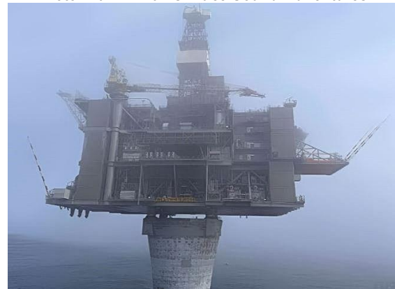
West White Rose - finally installed together, the Topside was mated to its CGS, and of course, it wouldn't be proper without Grand Banks fog!
