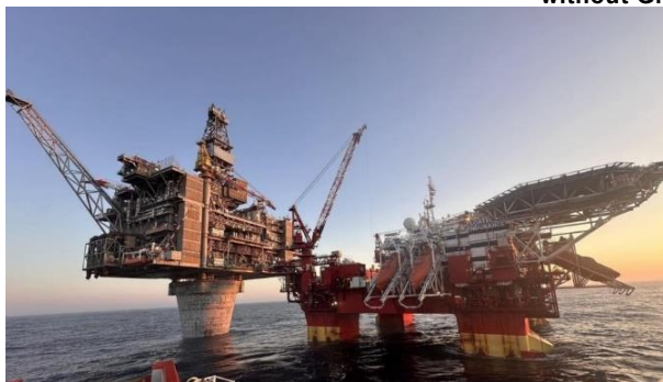
Floatel Endurance with focus shifting to the final stages of the project with the hook up and commissioning of the platform and the subsea tie-in work.
