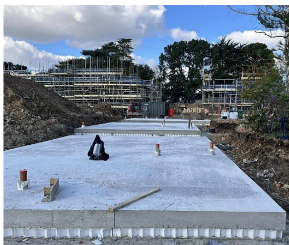
Building work seems to be progressing well. The refurbishment etc of Shackleton looks to be about to start soon as people can be seen working inside.
