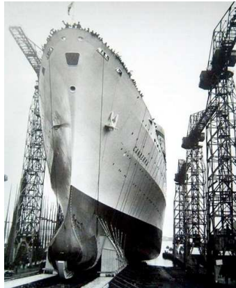
Canberra slowly sliding down the slipway
