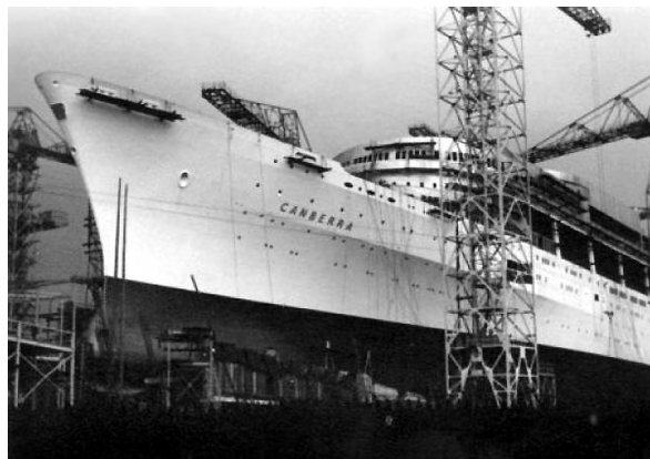
Canberra in the Harland & Wolff stocks whilst getting ready for launching
