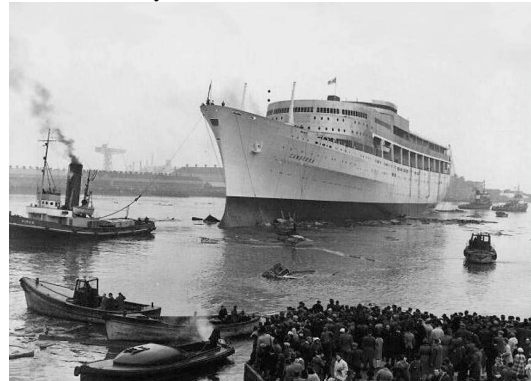
Finally the superb liner is in the water and ready to be towed to her fit-our berth
